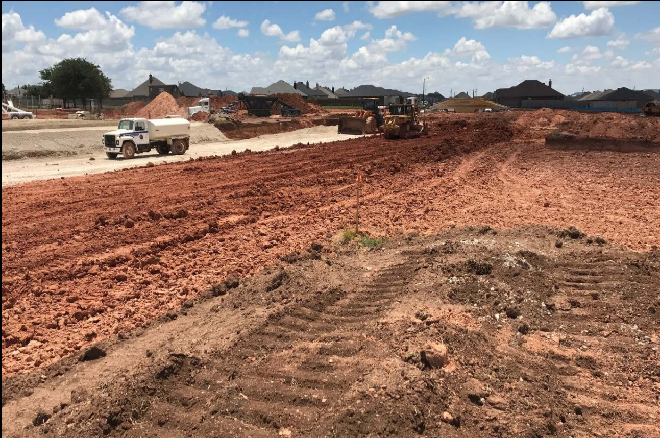
Placing Select Fill Material
