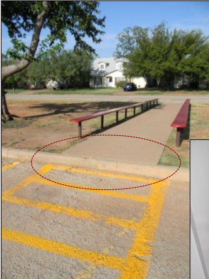
Missing ADA ramps at required accessible routes
