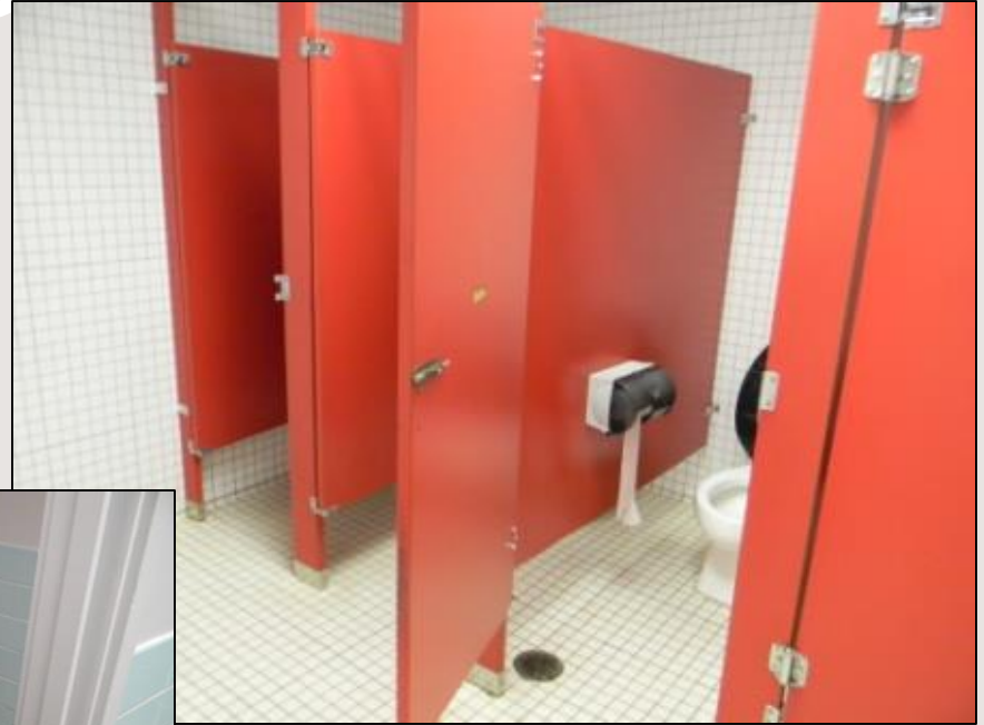
Non-ADA compliant toilet stalls, hardware and door swings
