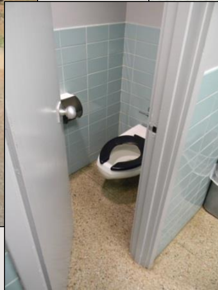
Non-ADA compliant toilet stalls, hardware and door swings
